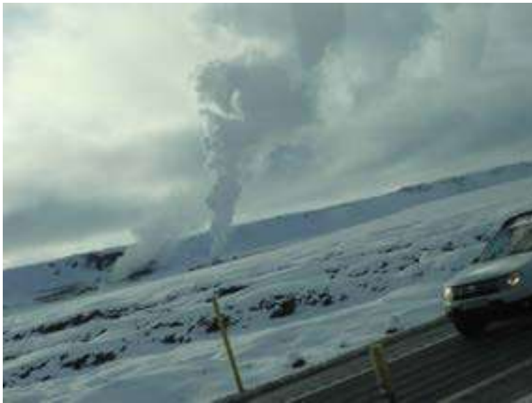
A geothermal power plant
